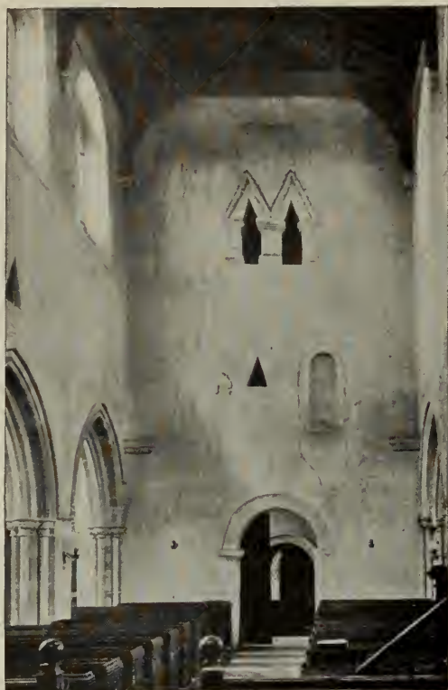
86. INTERIOR OF DEERHURST TOWER
